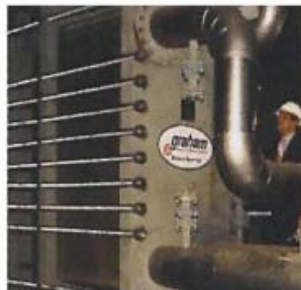
Plate heat exchangers
