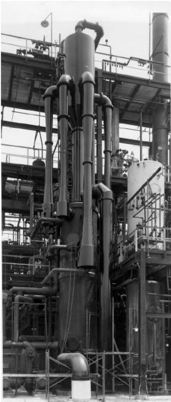
**Figure 5. Steam Vacuum Refrigeration Unit**
