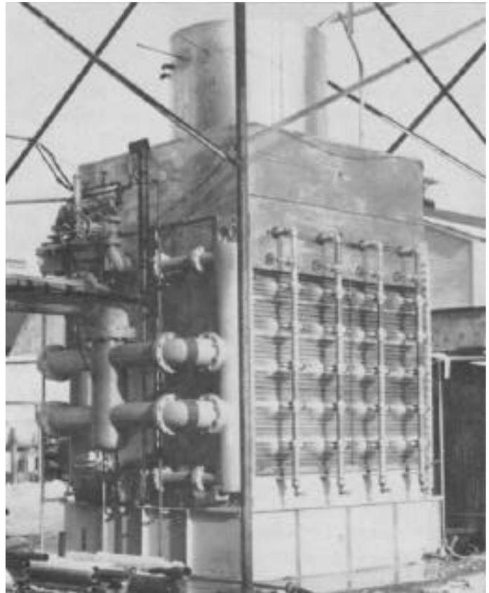
**FIGURE 1**-Evaporative cooled heat exchanger is in service as vacuum steam condenser. It contains 1,500 square feet of surface and handles 3,490 pounds of steam per hour at 2.0 inches mercury absolute pressure. Ambient wet bulb temperature is 70° F.
