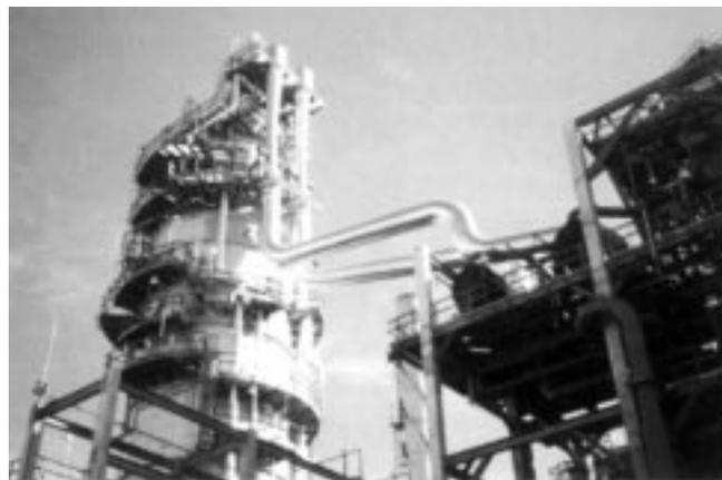
*Fig. 1. Twin-element, three-stage ejector system on crude vacuum tower.*
