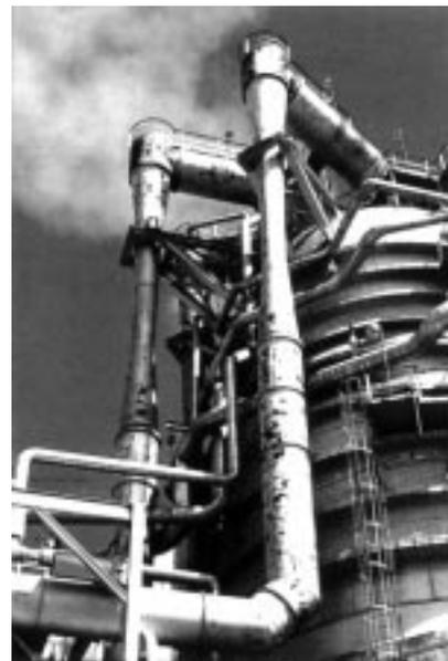
*Recently installed 1st stage ejectors included as part of a four stage ejector system serving a CVDU in Asia.*
