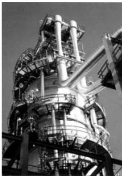
*Recently installed 1st stage ejectors included as part of a four stage ejector system serving a CVDU in Asia.*
