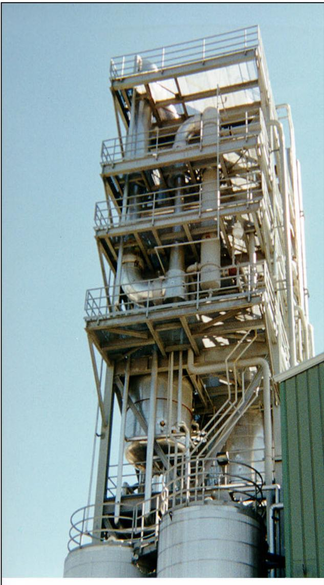
Figure 1. Ejector System for soybean oil deodorizer
