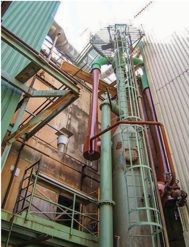
FIG. 5. OEM replacement ejectors on an SVRU.
